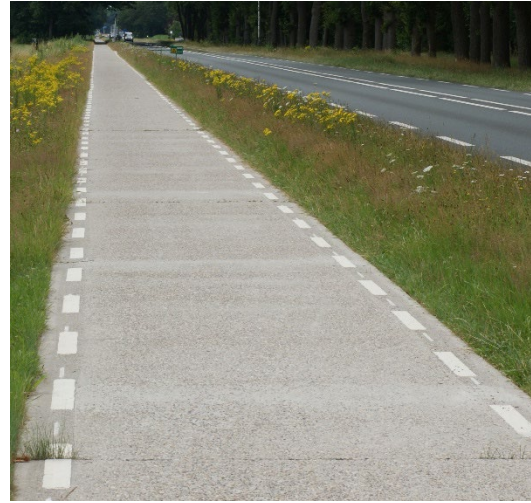
Figure 25 Surface with scaling in 2022
