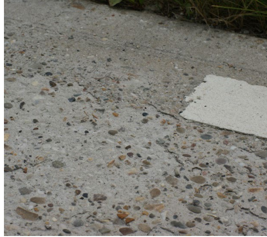
Figure 31 Progressive scaling Deventer-Holten
