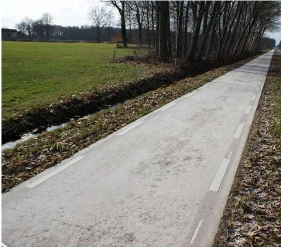
Figure 24 Surface with scaling in 2021
