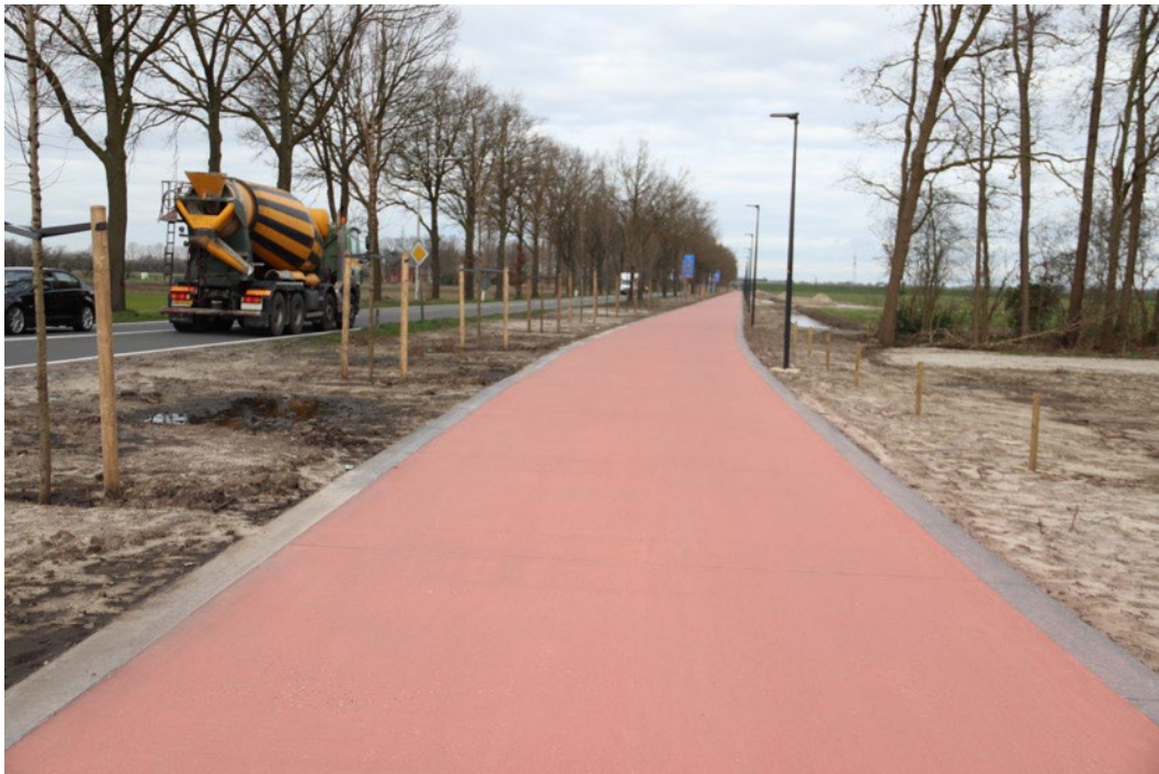
Figure 15 Overview of the bicycle path in March 2020
