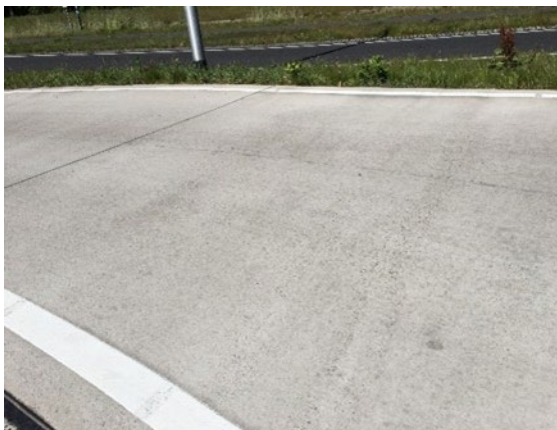
Figure 7 Main road surface in 2019
