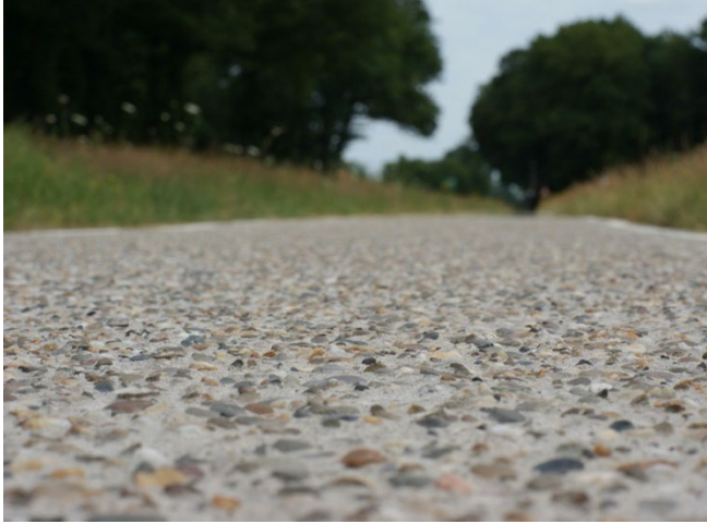
Figure 30 Surface texture surface Deventer-Holten
