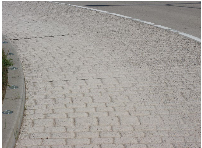
Figure 12 Truck apron in 2022
