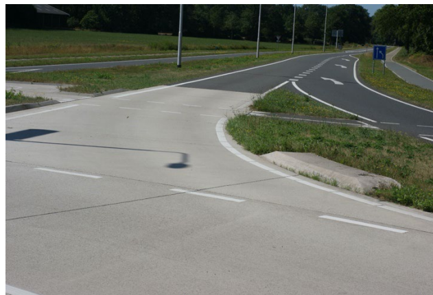
Figure 8 Main road surface in 2019
