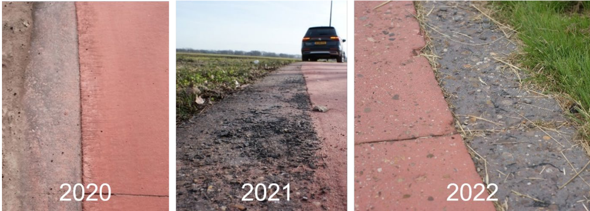
Figure 19 Scaling of the kerbs on the lower side in time
