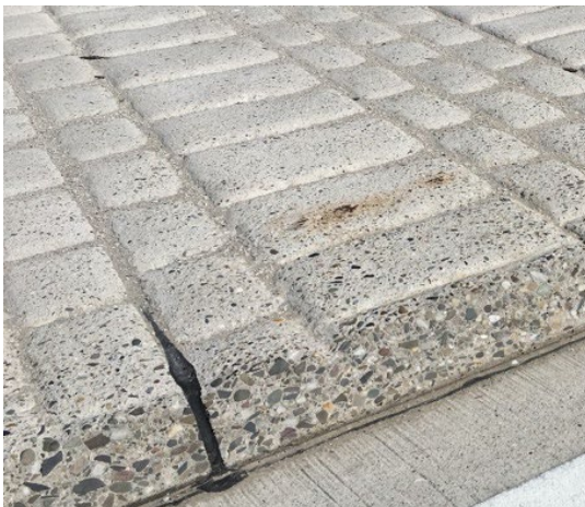
Figure 13 Truck Apron in 2019
