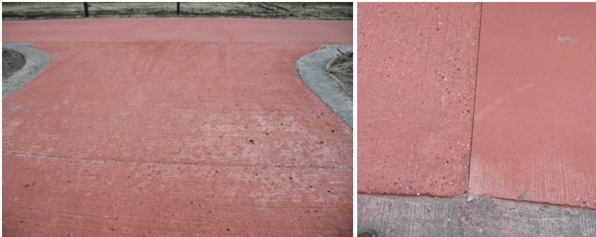
Figure 16 Difference between slipform paved and manual constructed (2020)
