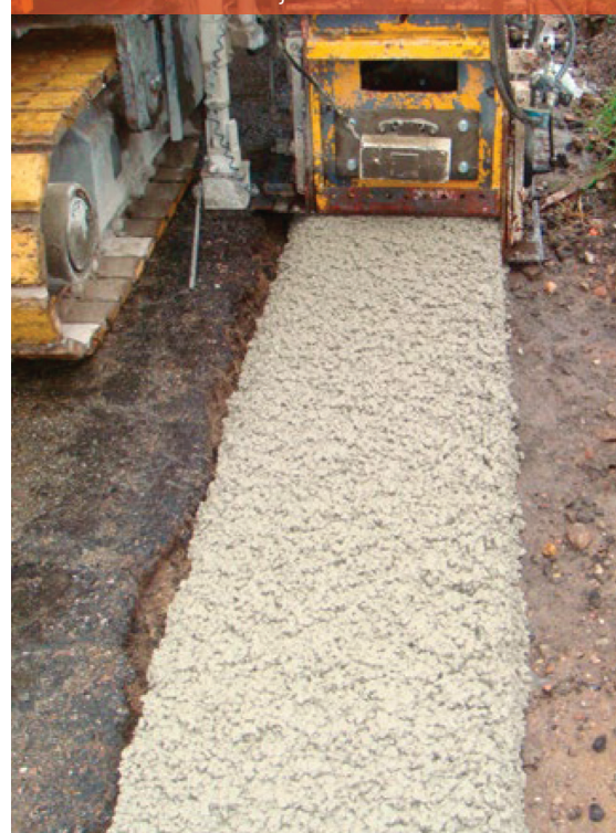
Construction of 'Bermcrete' in the Netherlands © Heijmans
